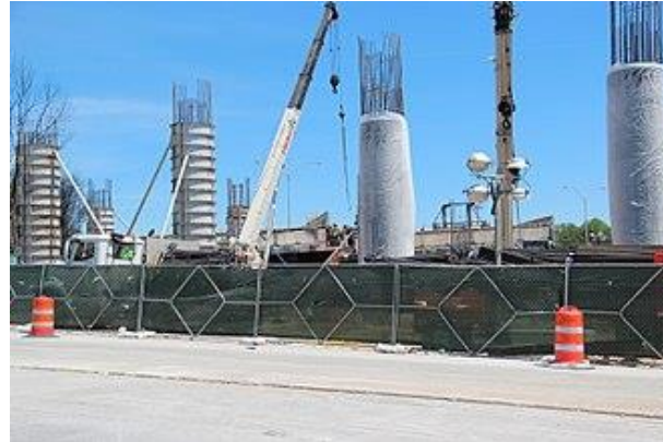
America, 2017. Fire cause bridge collapse
