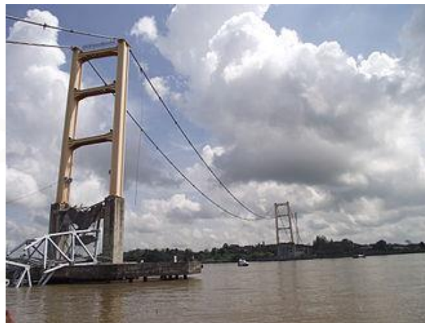
Indonesia, 2011. Repairing error cause deck destroyed
