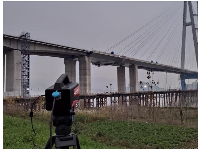
Wuxue Yangtze River Bridge
