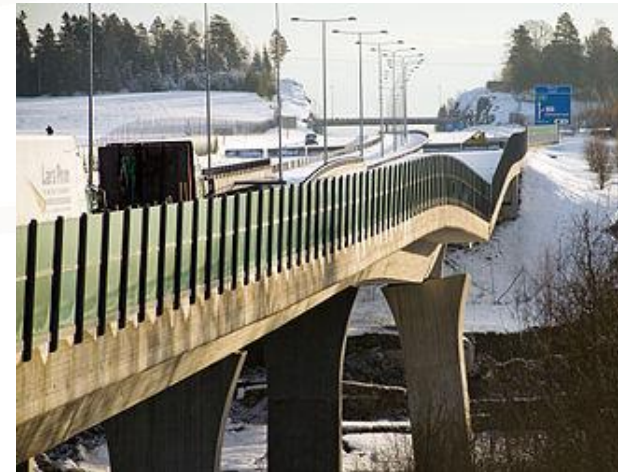
Norway, 2015. Landslide cause bridge collapse
