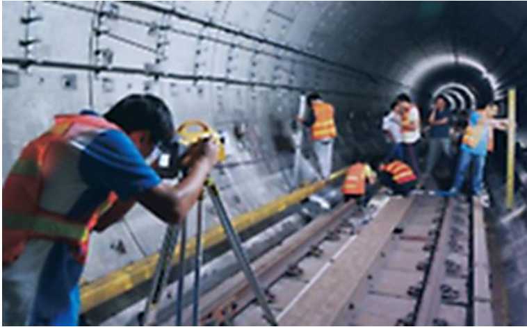
Total station and Level
